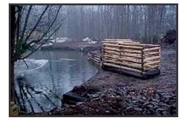
6) Timber rock crib being installed in Kingsford, Mississippi by the Pine Creek Watershed Conservation Project. High quality construction would be essential to placement of this style of rock crib within the Shearstown Estuary to withstand ice and winter storm conditions. Design may have to be modified to deal with specific conditions existing within the estuary.
